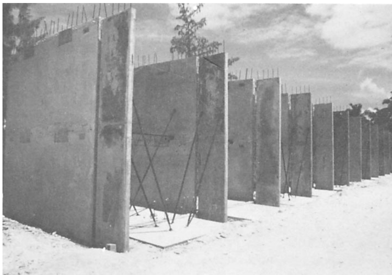
Figure 6-10.-Precast panels in position.
