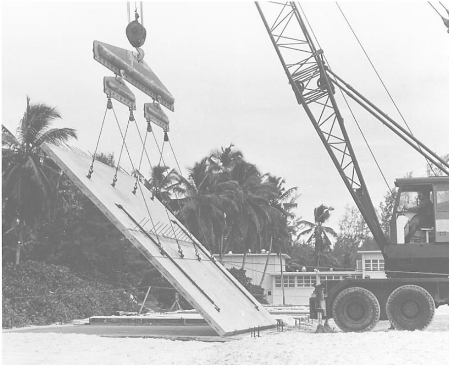
Figure 6-9.-Precast panels being erected by use of crane and spreader bars.
