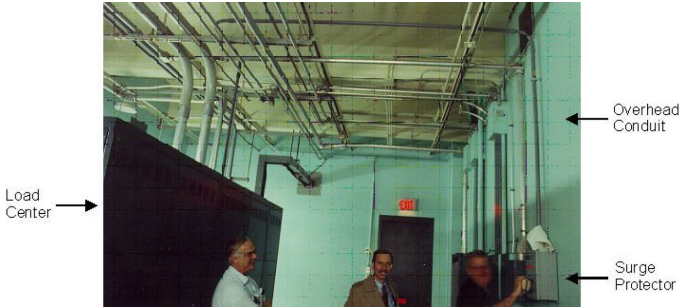
Figure 11-5. Less-Than-Optimal Installation by Including Safety Switch
