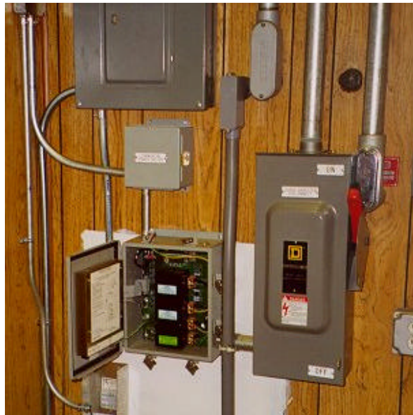
Figure 11-5. Less-Than-Optimal Installation by Including Safety Switch
