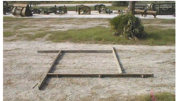
Figure 3-1. Metal Forms Set Up For A Square Floor Slab.
