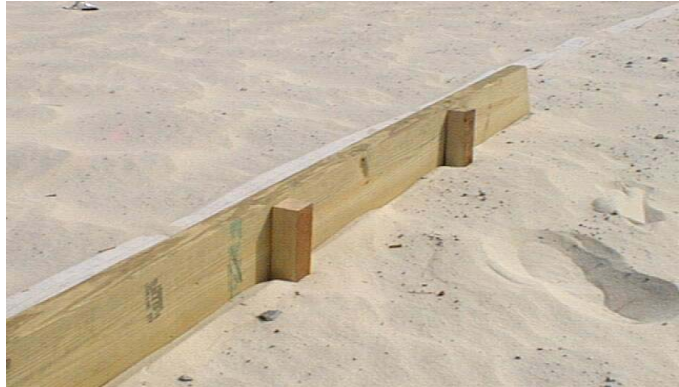
Figure 3-4. Wood Stakes with Wood Form.
